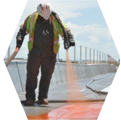
Roads and bridges Carreteras y puentes
